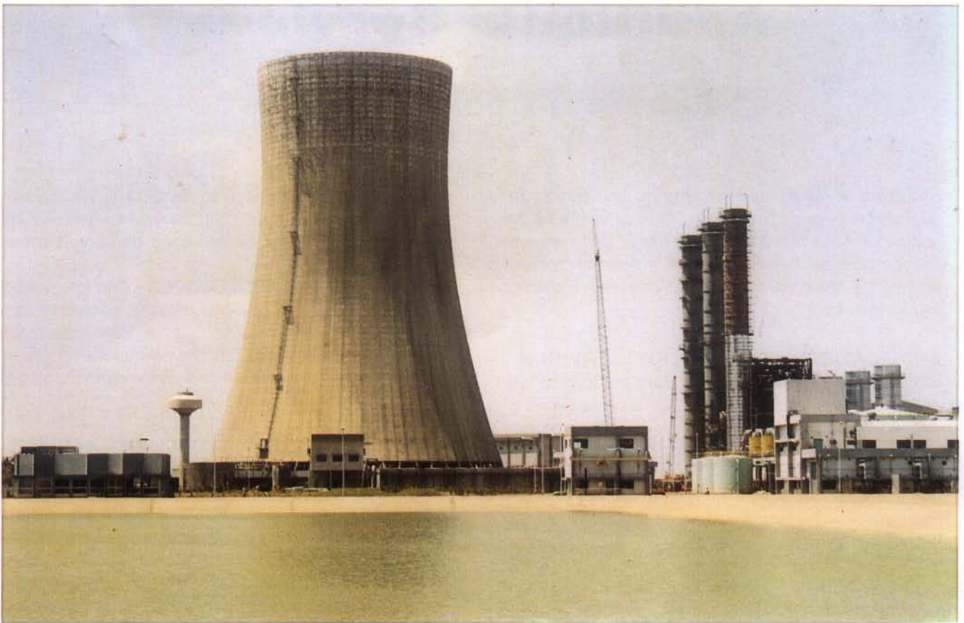
A Paharpur Class 800 Natural Draught Cooling Tower at Gujarat Torrent Energy Corp. Ltd's 655 MW Combined Cycle Power Plant at Paguthan. EPC Contractor - Siemens Ltd., Germany.
